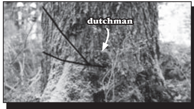
Figure 4-24—When the sloping cut and the horizontal cut do not meet exactly, a dutchman is formed. This kerf-wide cut makes the direction of the tree's fall harder to predict. It can also cause the tree to barber chair, lifting the log off the stump and placing the sawyer at great risk.
